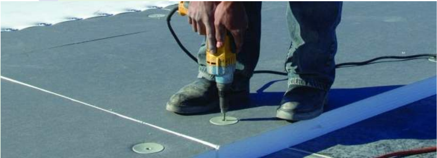
FIGURE 2B: INSULATION BOARD FASTENING SYSTEM
